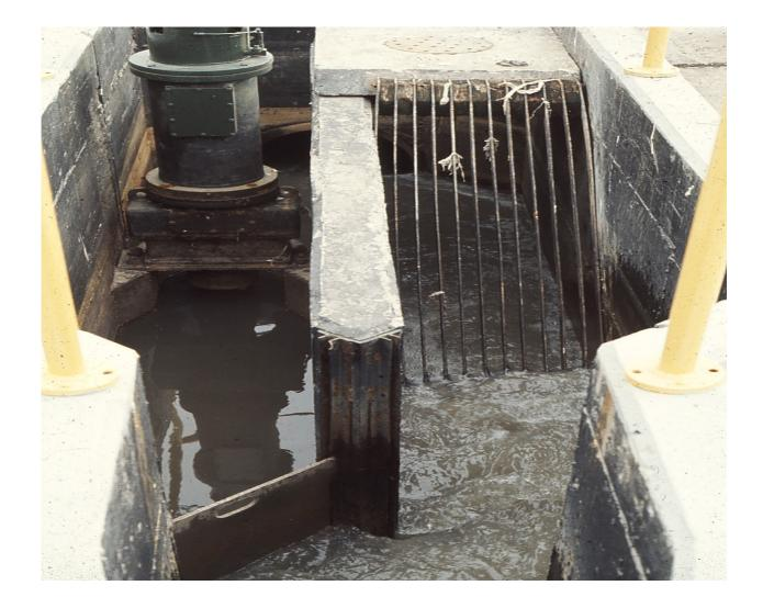
Velocity controlled grit chamber. Left chamber in service. Right chamber out of service.
